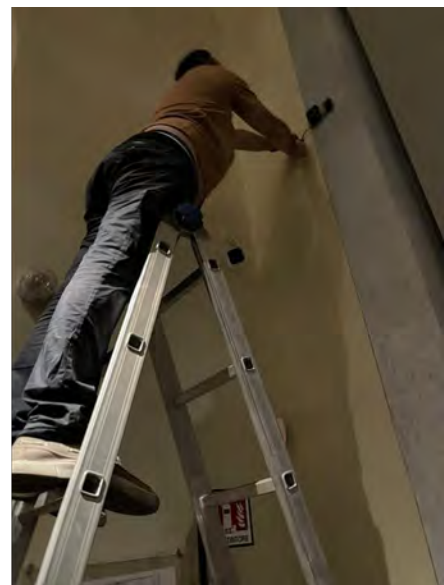
Figure 6. Workstation used for monitoring and data collection ( left ). Installation of UWB anchors on the walls to align with LiDAR-determined coordinates ( right ).
