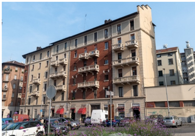
Figure 4. Picture of the case study building.
