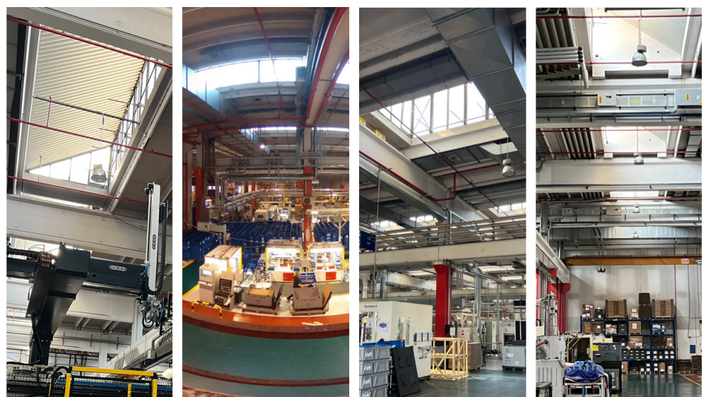
Figure 10. Technical survey of the industrial plant used to support the digital modelling and energy analysis process.
