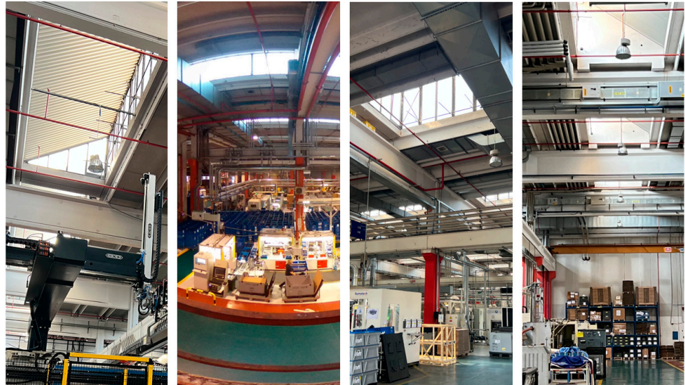
Figure 10. Technical survey of the industrial plant used to support the digital modelling and energy analysis process.
