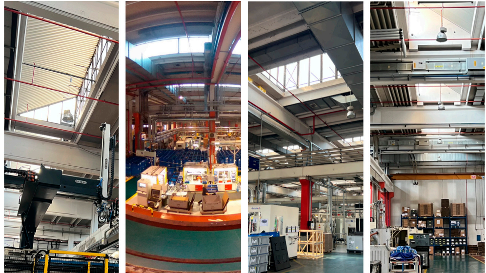
Figure 10. Technical survey of the industrial plant used to support the digital modelling and energy analysis process.
