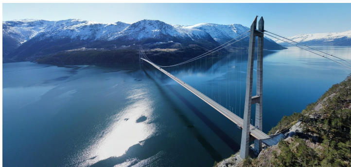
Figure 1: Geographical localization of the case study, and photo of the Hardanger Bridge courtesy of Nico West from Pixabay.
