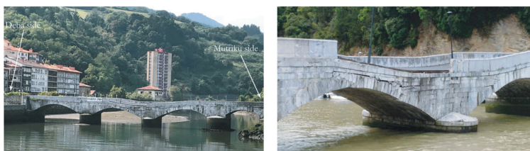
Figure 2. Deba bridge, Spain. The settlement of the central pier was induced by shipworm infestation in the timber foundation piles, from Malena et al. (2021).
