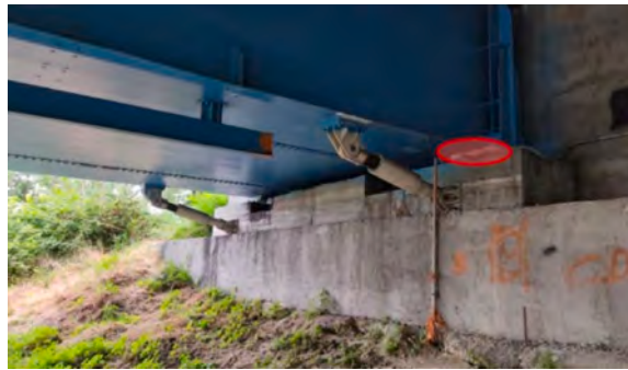
Fig. 4. Unidirectional longitudinal bearing at abutment 1.
