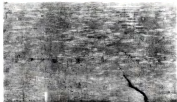
Figure 10. thermogram showing structural materials behind Vasari's Battle of Marciano
