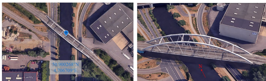
Fig. 1 Google earth view of the KW51 railway bridge
