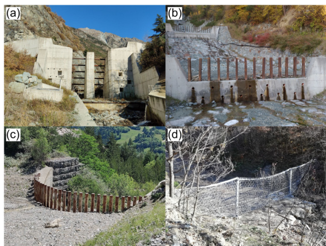
Fig. 1. Examples of typical barriers installed in areas prone to debris flows: (a) slit dam, (b, c) filter barriers, and (d) cable-net barrier.
