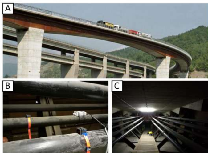
Fig. 2. A) Aerial view of the viaduct under analysis. B) Sensor positioning on prestressing cables. C) Prestressing cables.
