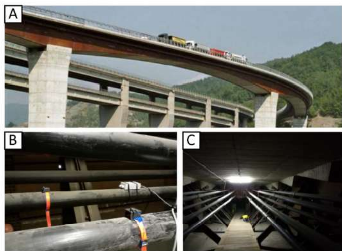
Fig. 2. A) Aerial view of the viaduct under analysis. B) Sensor positioning on prestressing cables. C) Prestressing cables.
