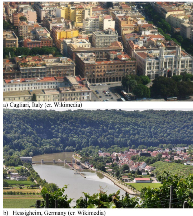
Figure 2. Comparison between the Cagliari city centre (a) and the Hessigheim (b) settlements' morphologies. From the aerial photographs, it is possible to observe the important differences between the two urban configurations in density and construction typologies. This difference reflects the available digital data.
