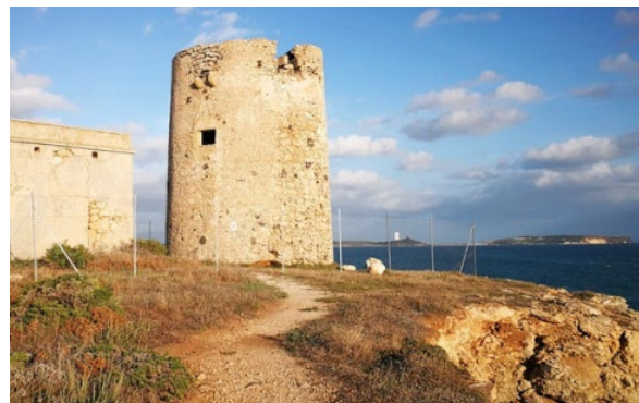
Figure 1. Sevo Tower. Cabras, Italy (cr. fortificazioni.net).
