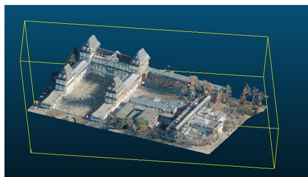
Figure 3: Pre-processed point cloud from aerial photogrammetry
