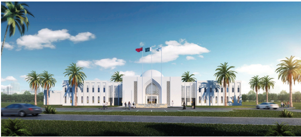
Figure 6. Pakistan–China Friendship Vocational and Training Institute rendering representing an eclectic architecture Source: Document from Gwadar Port Authority (GDA) office. Image used with permission from GPA, Copyright © 2025, GPA.
