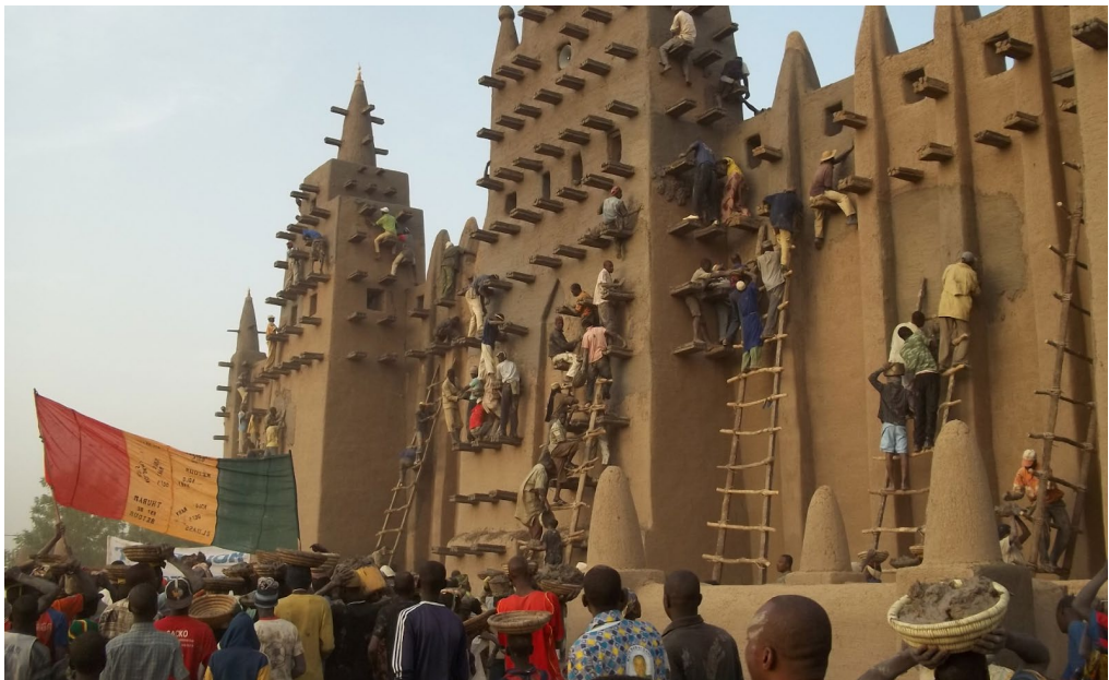
Fig. 1 – Replastering of Djenné mosque by the community in 2012 (Mission Culturelle de Djenné, F. Yamoussa).
