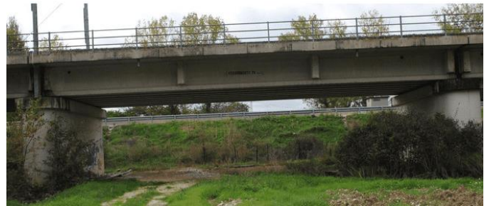
Figure 1: View of a typical span of the railway viaduct.
