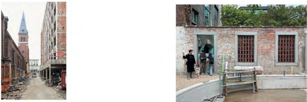
Figure 10. Left: Freeing the church of the added storage volumes gives some air to the public garden-to-be and allows for a strip of fertile soil; Right: Reinforced concrete beams are disguised as garden elements such as a pond, stairs and a bench, creating the possibility for heavier loads (greenery). (©ono architectuur).
