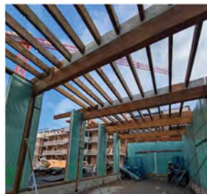
Figure 5. Timber construction with only reused beams.
