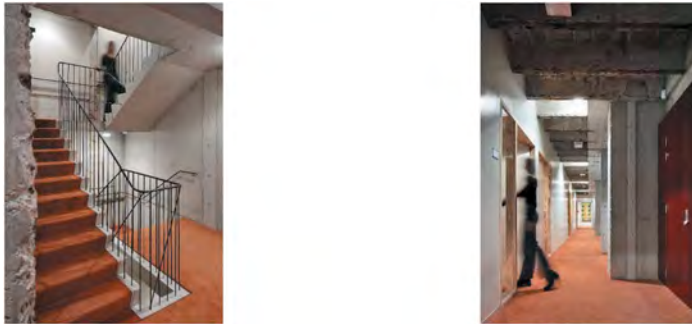
Figure 9. An adaptation of the lower levels of the staircase (left) leads to additional steel strips, embracing the central core (right) with elevator and stairs. (©Filip Dujardin).
