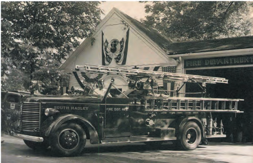
Figure 1. Historic Photo of the Phoenix as an active Fire Station.
