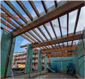
Figure 5. Timber construction with only reused beams.
