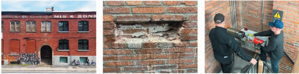
Figures 1, 2, 3. An existing building at 3558 Saint Patrick Street, Montreal, was selected as a case-study and used to collect detailed information on material and construction systems.
