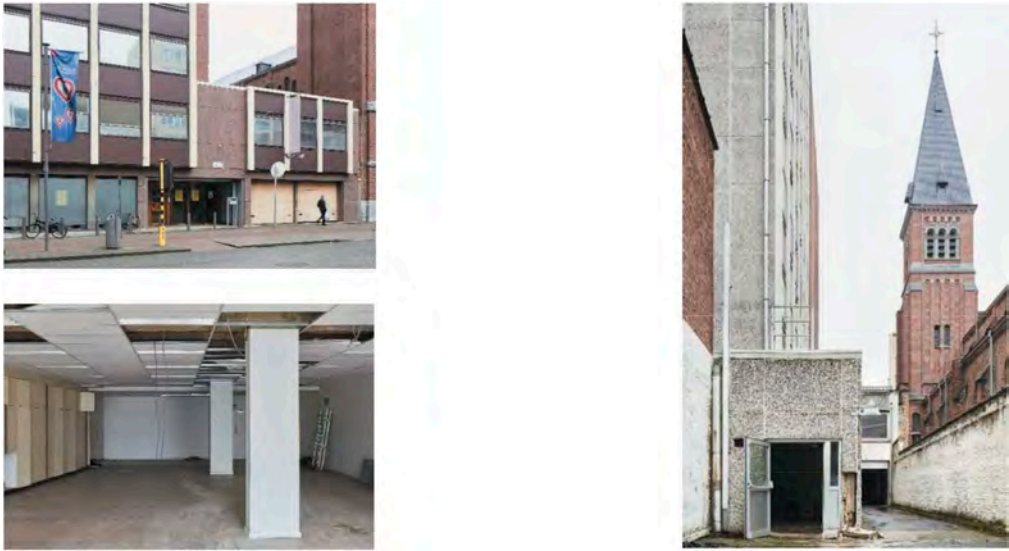
Figure 1. Top left: At M127, a '60s office building behaved hermetically towards its surroundings; Bottom left: The concrete structure was hidden behind wafer-thin coverings. Daylight hardly entered in the deep ground floor level; Right: The outdoor space was fully asphalted and intended for access with vehicles. The only strip without parking underneath was filled with storage volumes from the adjacent church. (©ono architectuur).
