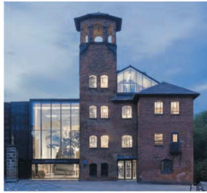
Figure 4. Museum of Making, Derby (GCA Consulting Engineers).
