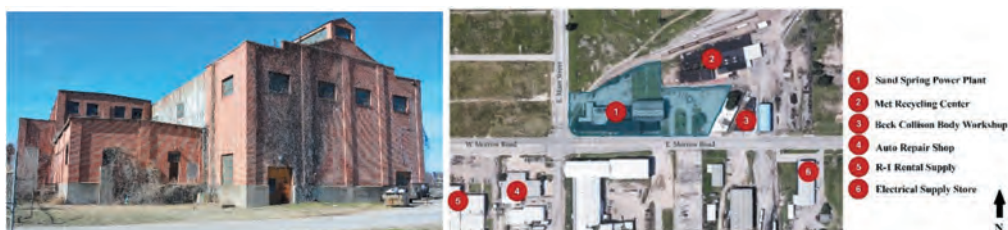
Figure 1. Sand Springs power plant (Photo by authors) Figure 2. Site context, graphical representation, Google Earth.
