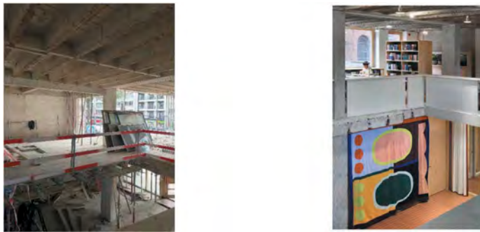
Figure 7. Left: Low stacked floors are cut away at precise locations at ground floor; Right: New cuts through the building are left in their raw state. (©ono architectuur, Filip Dujardin).
