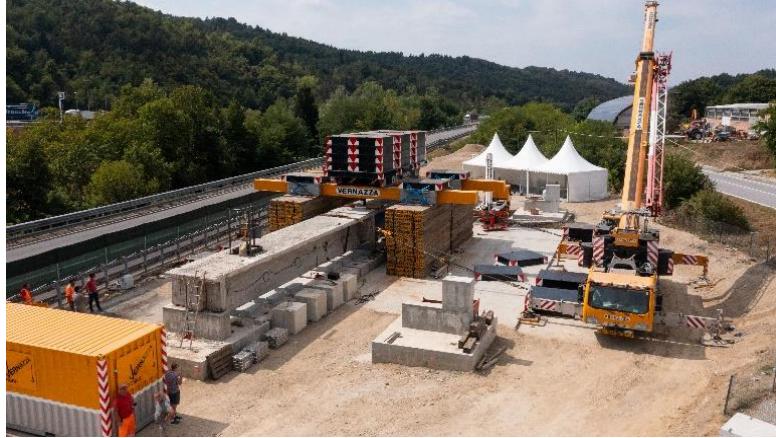
Fig. 4. Ultimate test layout arrangement featuring the 3000 kN counteracting structure.
