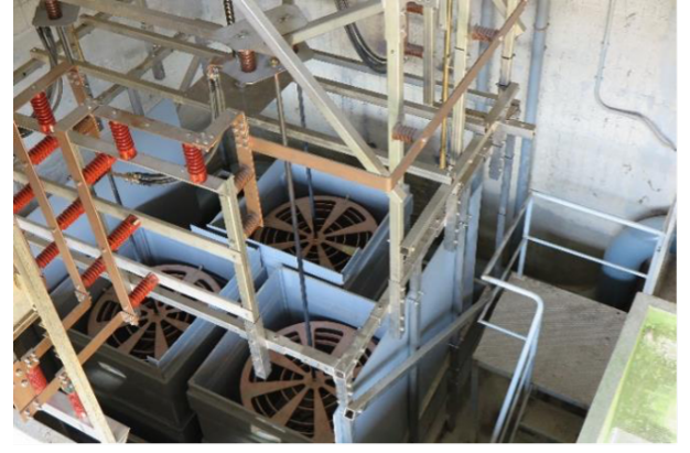
Fig. 3: New design of the power dissipation system.
