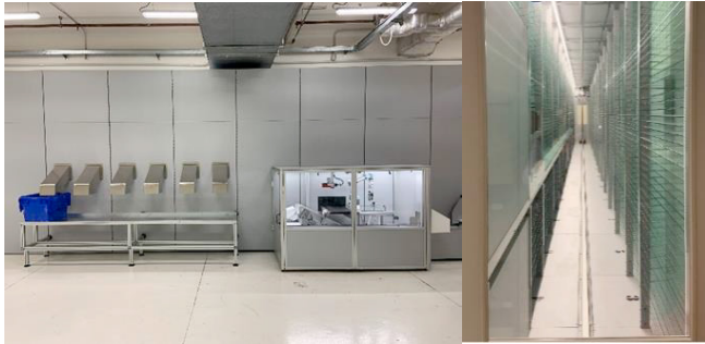
Figure 1. Automated Miniload storage system
