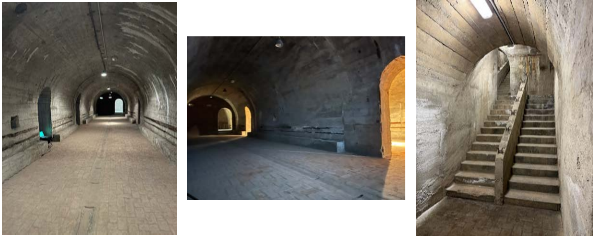
Fig. 11 Example of typical underground cavities used for air shelters and currently abandoned.
