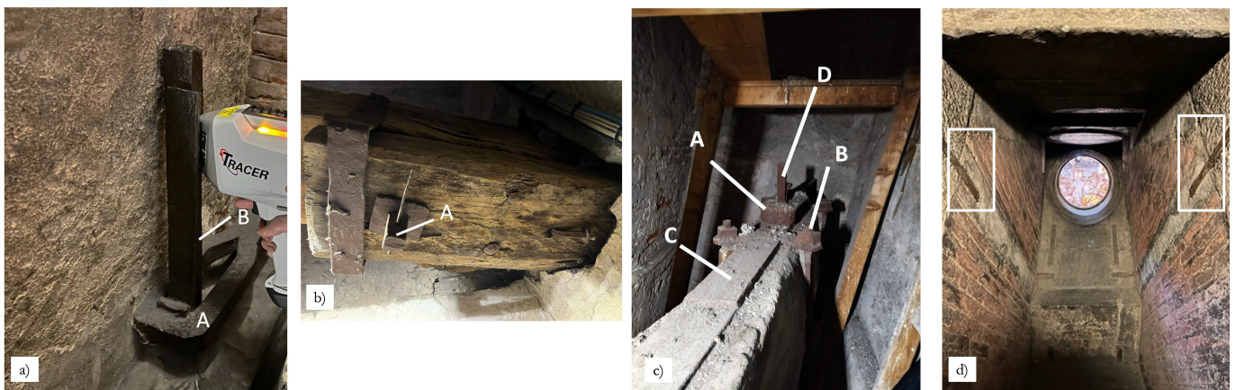
Figure 3. a) Metallic joint in compartment 8; b) Chestnut chain and metallic joint in compartment 12; c) Chestnut chain and metallic joint in compartment 16. The white letters indicate the areas of analysis; d) Compartment and the two metallic rods on the sides (white rectangles).
