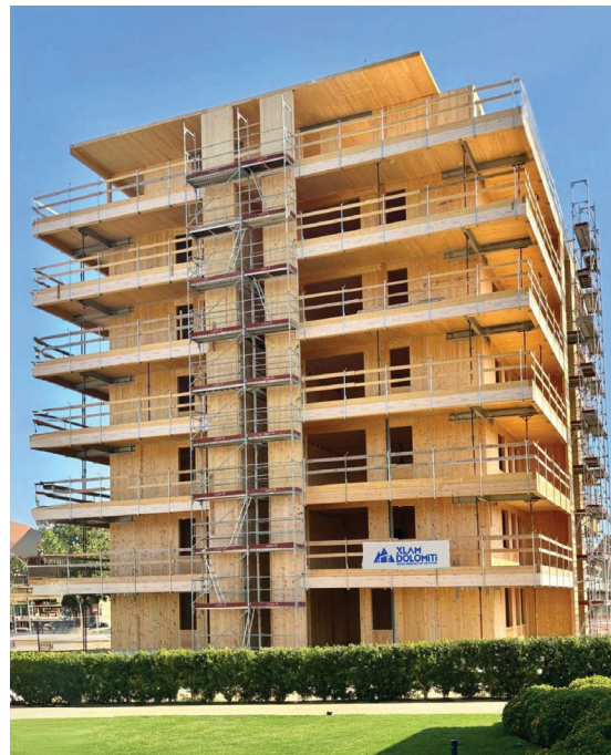
Figure 3: Construction site of XLAM Dolomiti in Italy.
