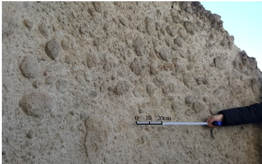
Fig. 3 A view from side wall of Koimesis Tes Panagias Church presenting various size of andesite blocks welding in a fine-grained matrix.
