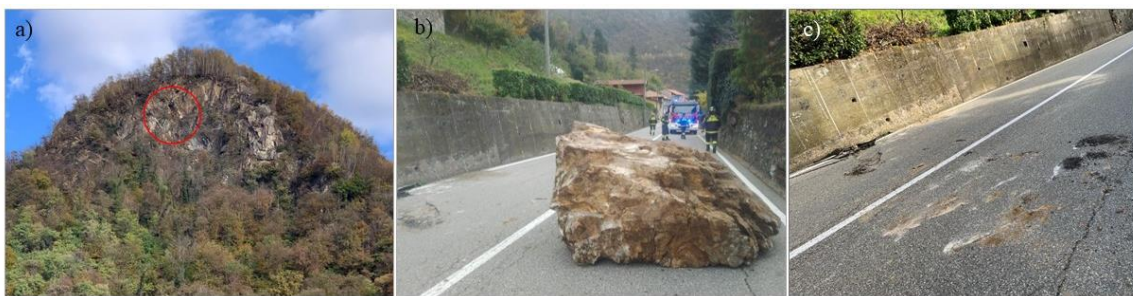
Fig. 2 a) detachment niche located on the Barbavara castle rock slope; b) kinzigite rock block of about 3 m 3 that detached in November 2023, hitting the road; c) road damaged by the rock collapse.
