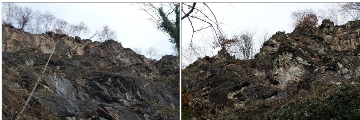
Fig. 3 Slope after rock removal.
