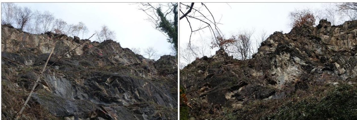
Fig. 3 Slope after rock removal.
