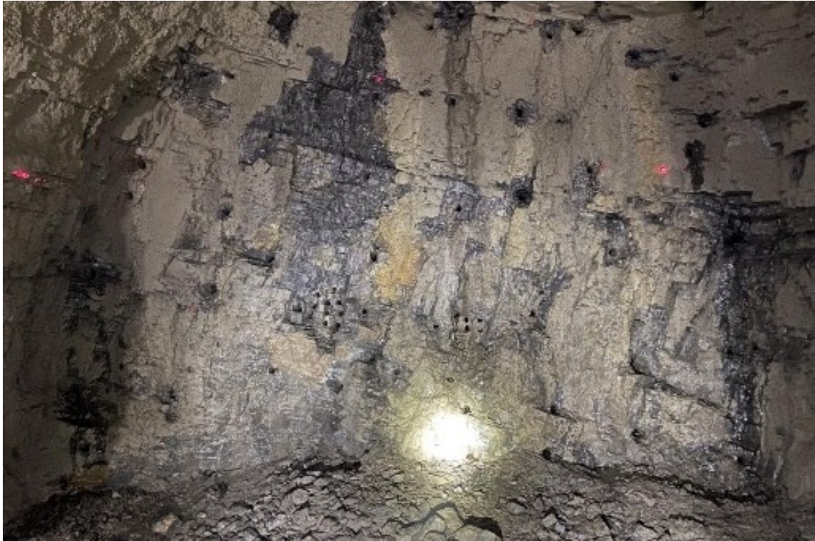
Fig. 3.4 Photo of a palm face in the tunnel to be tested
