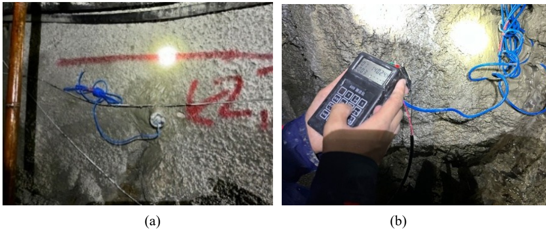
Fig. 7.3 Field arrangement and monitoring of multi-point displacement meter. (a) Field arrangement. (b) Field observation.
