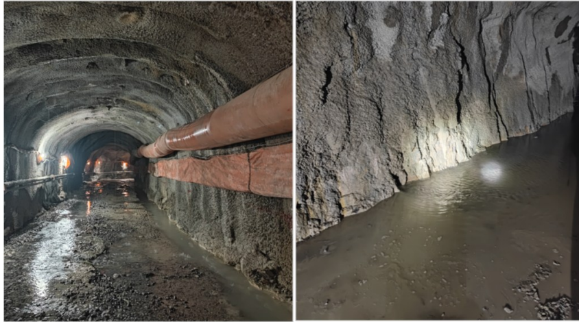
Fig. 1.2 A water-rich tunnel in Kunyang mine
