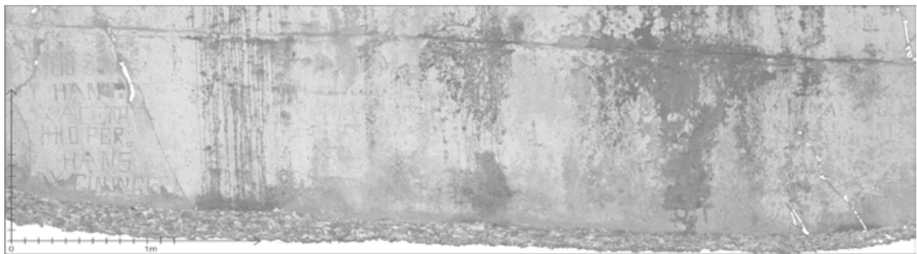
Figure 9. Orthophoto of an area of the 107 meters of stone walls of the Fingalshöhle, showcasing graffiti readable in the TLS-data (left and right), also visible are the moist areas in darker grey.
