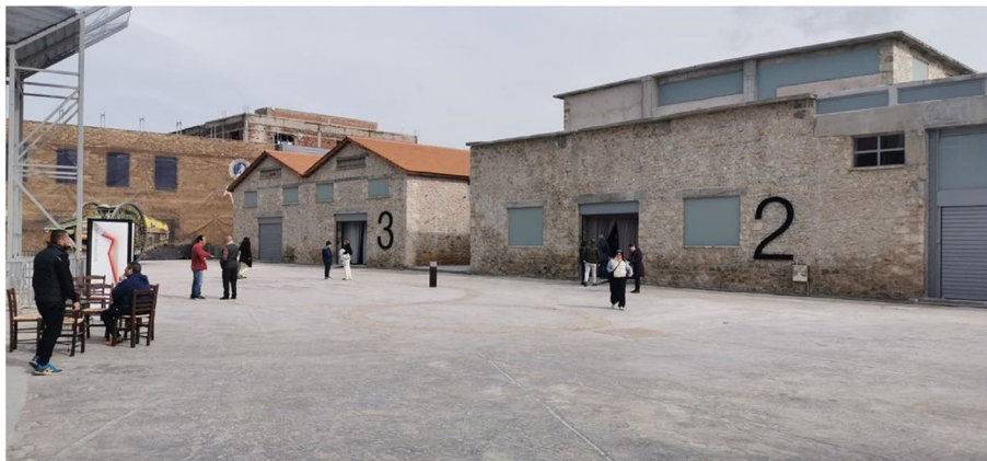
Fig. 7 Three specifically restored stone-built warehouses in the Old Olive Mill Factory complex in 2023
