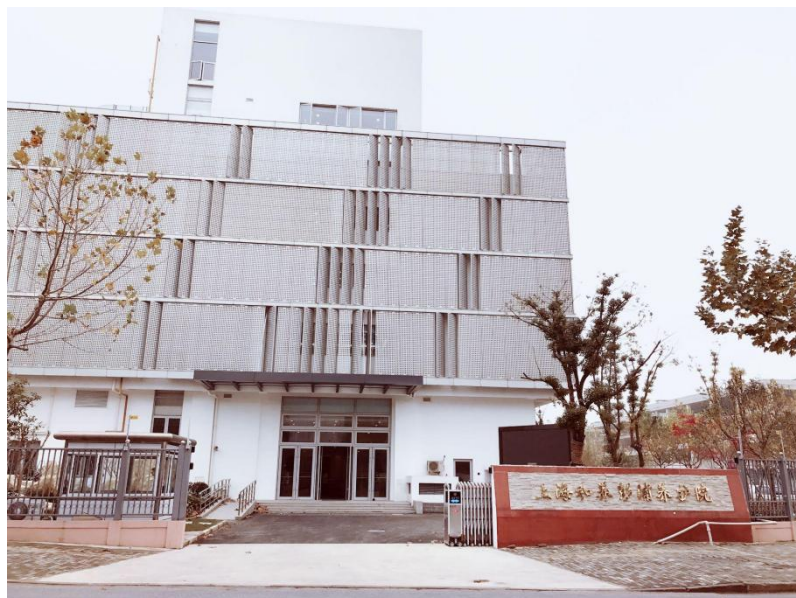
Figure 3. Shanghai Heyang Pengfu Pension Institution. Source: Shanghai Jingan District Civil Affairs Bureau.
