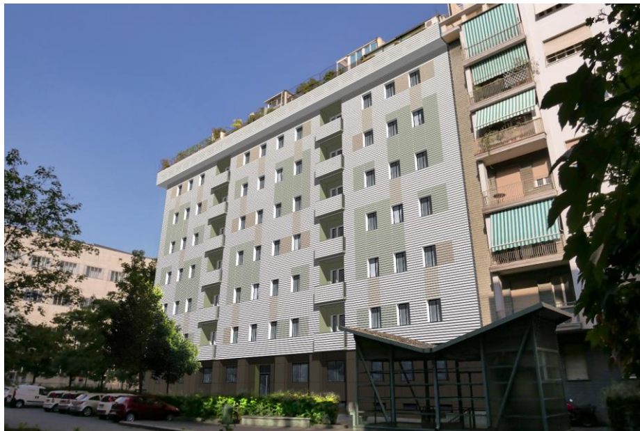
Fig. 7. Filigrana pattern on a residential multi-storey building (authors’ elaboration) © 2020, Paolo Piantanida, Antonio Vottari
