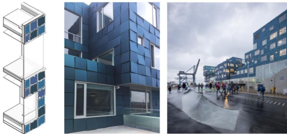
Fig. 3. Copenhagen International School (C.F. Moller Architects). Detail of the facade with BIPV solar modules © https://integratedpv.eurac.edu/en/case-studies/copenhagen-international-school.html
