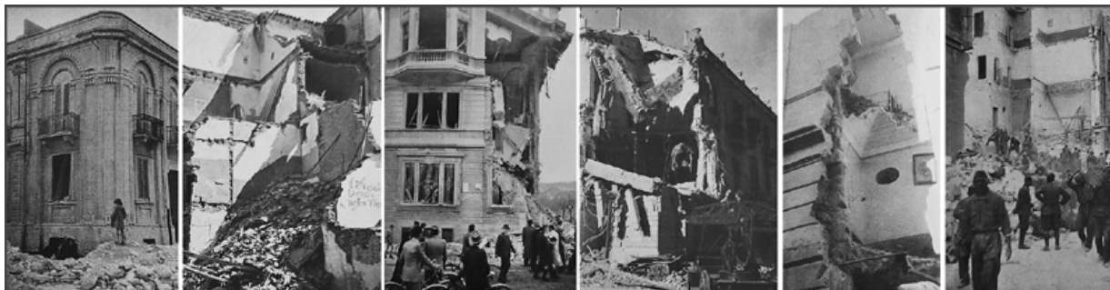
Fig. 2: Images portraying the damage that occurred to buildings with different types of construction. Issue 10 of Engineer of 1944, pp. 577-585.
