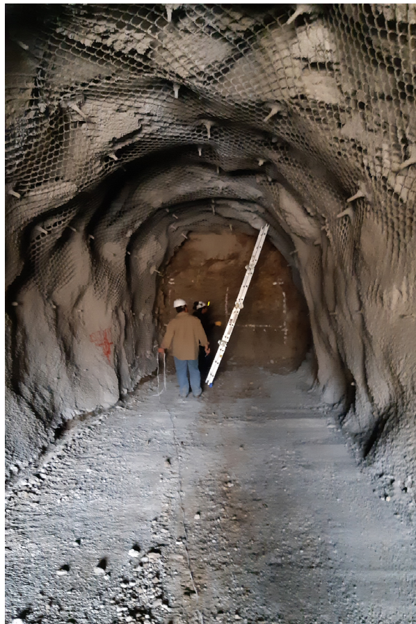
Figure 4. Inside view of the tunnel. The heads of the rock bolts are clearly visible on the vault of the tunnel.
