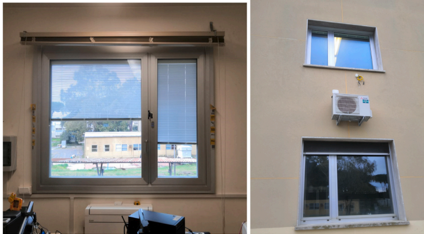
Fig. 3. Inside view of a W2 window with the solar shading device partially activated (left) and outside close-up of the facade, where the intrados of the windows are clearly visible.
