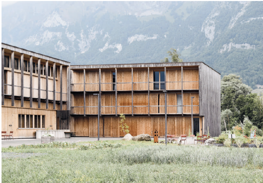
Fig. 2 | The Landwirtschaftliches Centre St. Gallen viewed from the inner courtyard. The image depicts the connection between the two-storey teaching wing and the three-storey dormitory wing (credit: the Authors, 2023).
