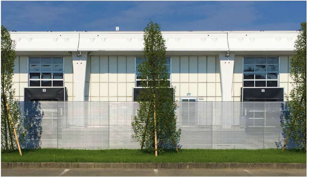
Figure 6. The Crema factory after the restoration by Ermentini Architetti, 2018. ©Ermentini Architetti
