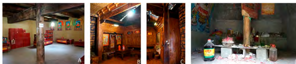
Figure 2. Different forms of central pillars (images from Qin FQ [13]). (A) Malcon Djokovic official residence; (B) Mosuo (female pillar); (C) Mosuo (male pillar); and (D) Tibetan central pillar of the lama pagoda.
