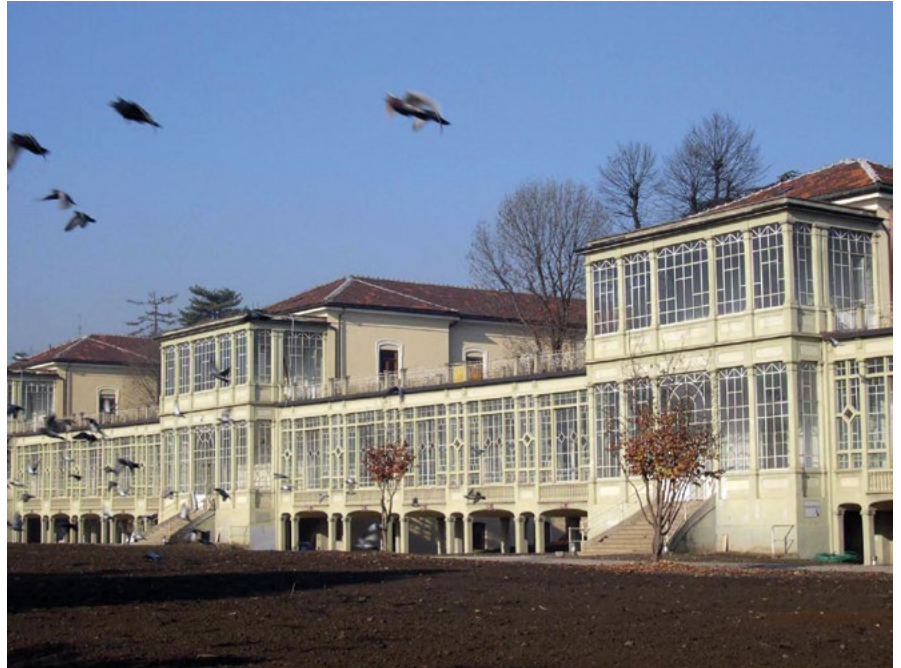
Fig. 12 – Former Riberi Hospital in Turin, the glass gallery and the central garden, after the restoration (2006)
