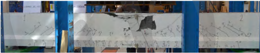
Fig. 4 Figure of the failure for beam 4 (LWAC65_20_100).
