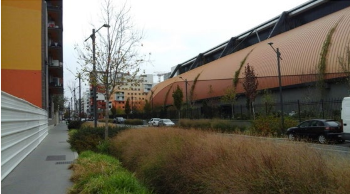
[FIG. 3] The factory CPCU in Saint-Ouen , ©Varvara Toura, 2023. The factory CPCU of the Parisian company of urban heating is located in the site of Docks-de-Seine near new residential buildings and shows the continuous presence of industrial activities in the area.
