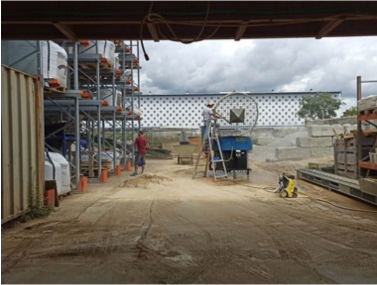
[FIG. 3] Saskia Gribling (2023). BC: the construction hall.
