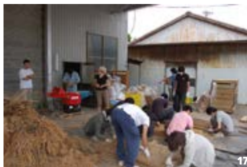
16. Extracting materials that can be reused from the demolition of a dozō in Wajima. Hagino Kiichiro 2007. 17. Cutting the old tatami straw into chops to be mixed with mud for plasters. Hagino Kiichiro 2007.
