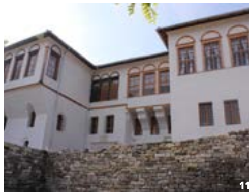
10-11. Restoration and revitalisation of Babameto House. On the left the situation in 2008; on the right the house in 2013 after the Gjirokastra Conservation and Development Organization (GCDO) and CHwB Albania joint restoration and revitalisation project. Gjirokastra Foundation GCDO and CHwB Albania. 2008, 2013.
