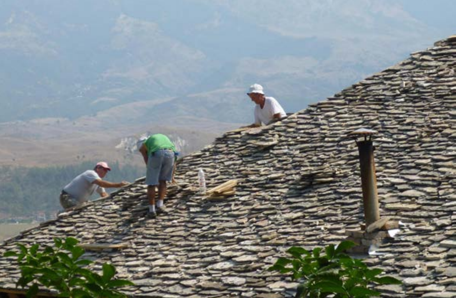
4. Stone roof restoration using traditional techniques in the frame of REVATO Project. Edvin Lamçe 2013.
