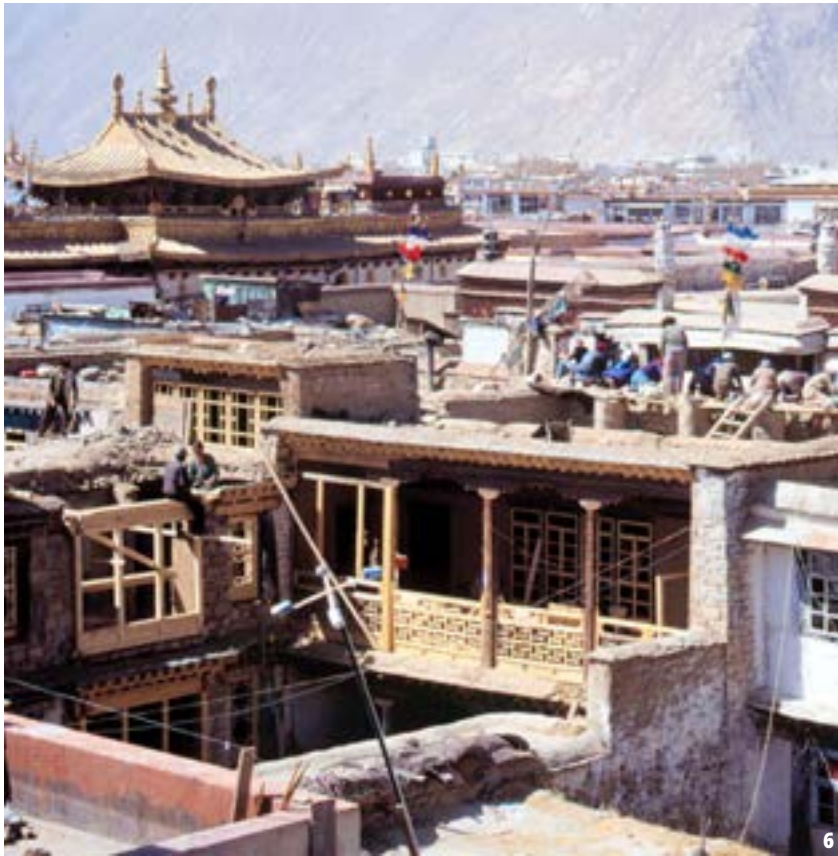
6. Restoration work of Rongdra House. Courtesy of Tibet Heritage Fund, André Alexander 1999.
