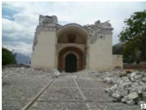
13-14. Temple of Ichupampa, before and after restoration. Ángel Guillén Archive 2009-2016.
