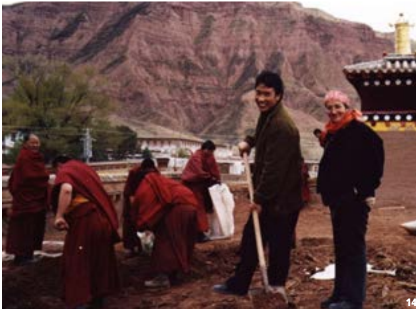
14. The monks disassembled the roof and carried the soil away so we could repair the structure. Courtesy of Tibet Heritage Fund, Lhundrup Dorje 2003. 15. After drying, people gilded the tsatsa statues and painted the eyes and mouth of the main statue's face on each one. Courtesy of Tibet Heritage Fund, Hirako Yutaka 2007.
