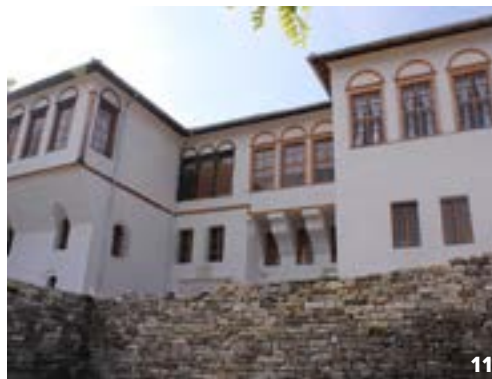
10-11. Restoration and revitalisation of Babameto House. On the left the situation in 2008; on the right the house in 2013 after the Gjirokastra Conservation and Development Organization (GCDO) and CHwB Albania joint restoration and revitalisation project. Gjirokastra Foundation GCDO and CHwB Albania. 2008, 2013.
