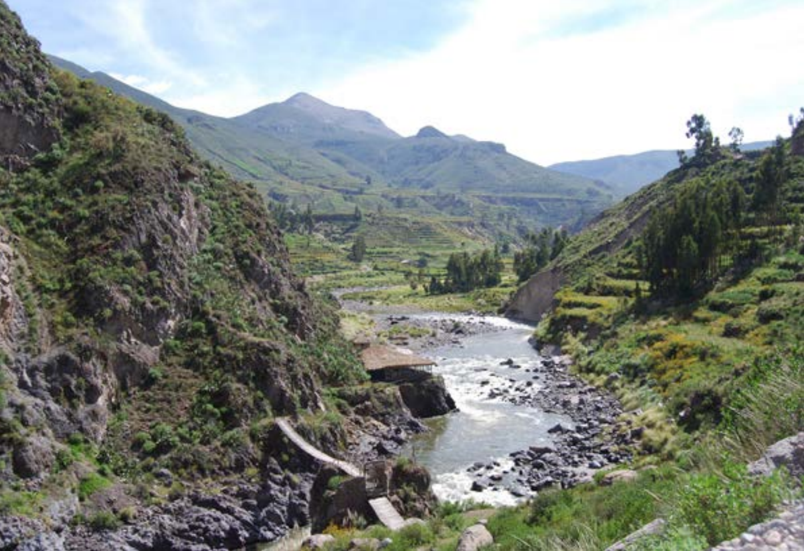
17. Connections between the banks of the Colca River in Yanque. Ángel Guillén Archive 2009.
