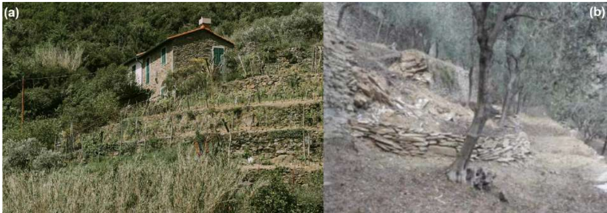
Fig.1: (a) Terrace in Liguria (Photo: Matteo Badani) ; (b) Shallow Landslide on Stone Terrace (Source: Giordan et al. (2017))
