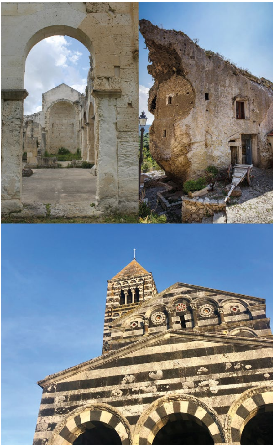
Fig. 2 – The case study of the GAL Anglona Coros area (Sardinia Region, Italy): Cultural Heritage of the winning circuit of the CA survey. Top right: Church of San Nicola di Sinis, Sedini (Source: Francesca Pasquino, April 2023). Top left: Domus de Janas, Sedini (Source: Francesca Pasquino, April 2023). Bottom: Basilica of Saccargia, Codrongianos (Source: Francesca Pasquino, January 2023).
