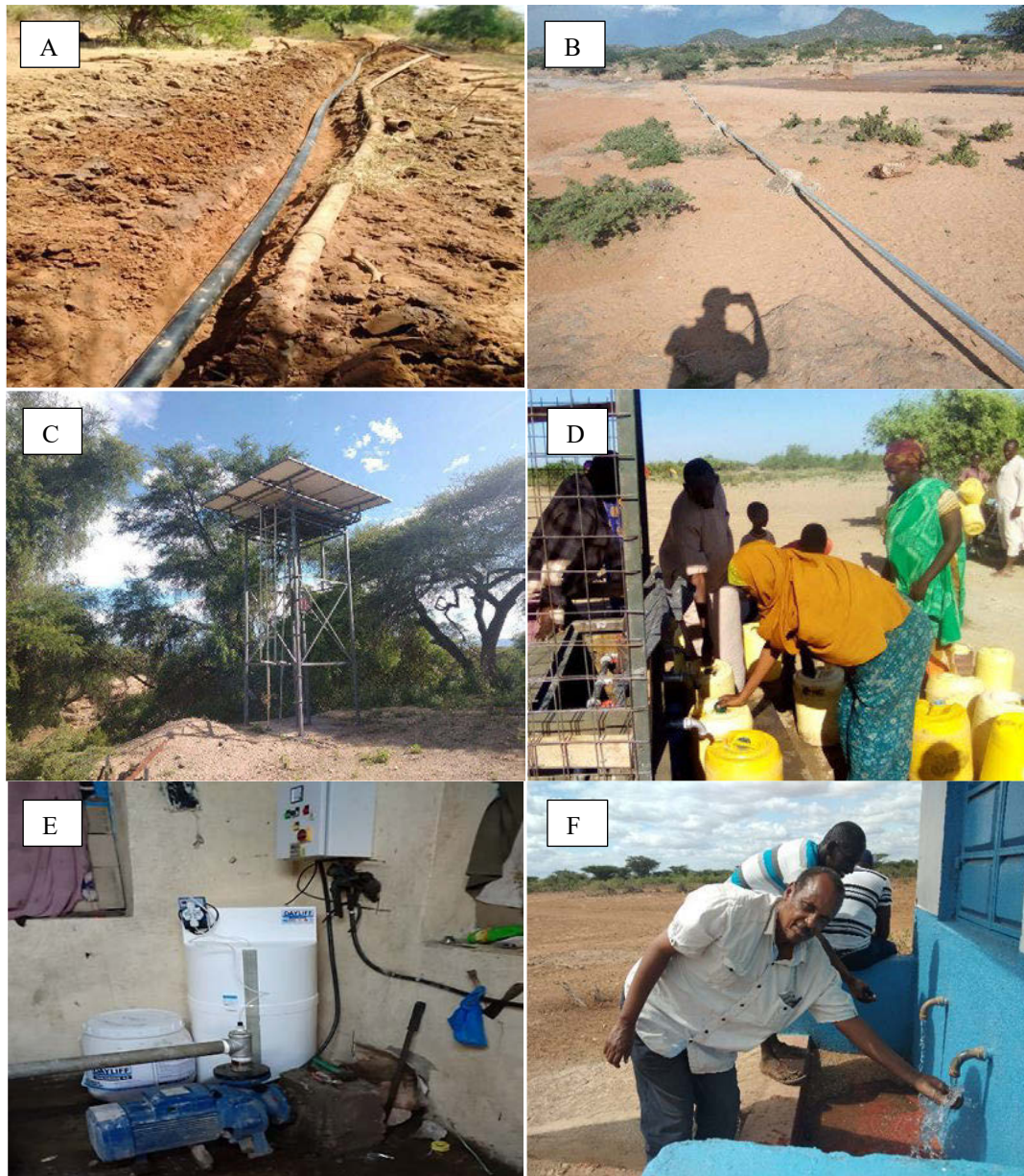
Figure 2. A) New installed HDPE pipes in the Bulesa village B) New pipeline in the Kipsing village. C) Borehole in the Kipsing Village with added solar panels for the new pumping system. D) Women fetching water at a community water point in Sericho village. E) Inline chlorine dosing equipment installed for Kinna village water supply system. F) The director of the water service during the launch of the new water kiosk in the Gafarsa village
