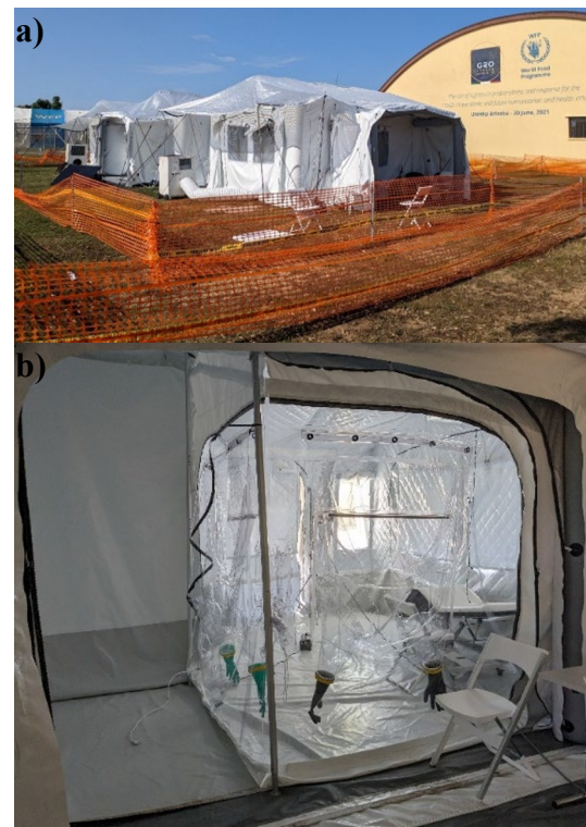
Fig. 1. a) The humanitarian tent installed in the testing camp of Brindisi. The installation results from assembling repeatable and symmetrical blocks, generating a multi-room environment. b) Each block has a confined area with a transparent layer, as shown at the bottom. The transparent layer acts as a barrier to separate the area where the patient rests (room #1) from the area devoted to the doctor's operation (room #2).
