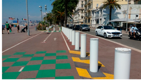
Figure 1. Example of vehicle security barriers (VSB) commonly used in an urban environment.
