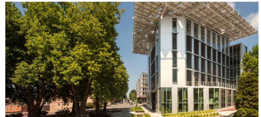
Bullitt Center, Seattle da: https://bullittcenter.org
