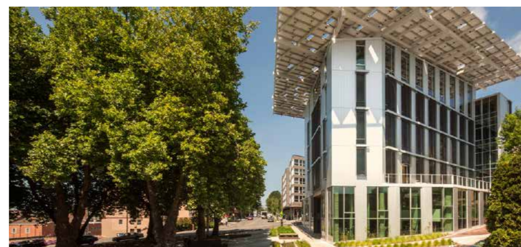
Bullitt Center, Seattle da: https://bullittcenter.org
