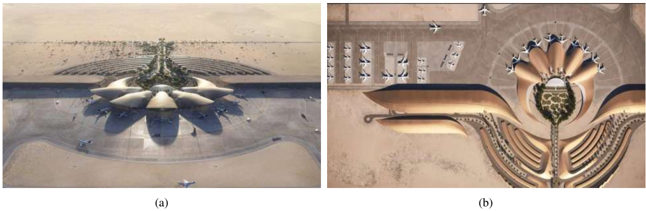
Fig. 6. Front (a) and top (b) view if the Red Sea International Airport [15].
